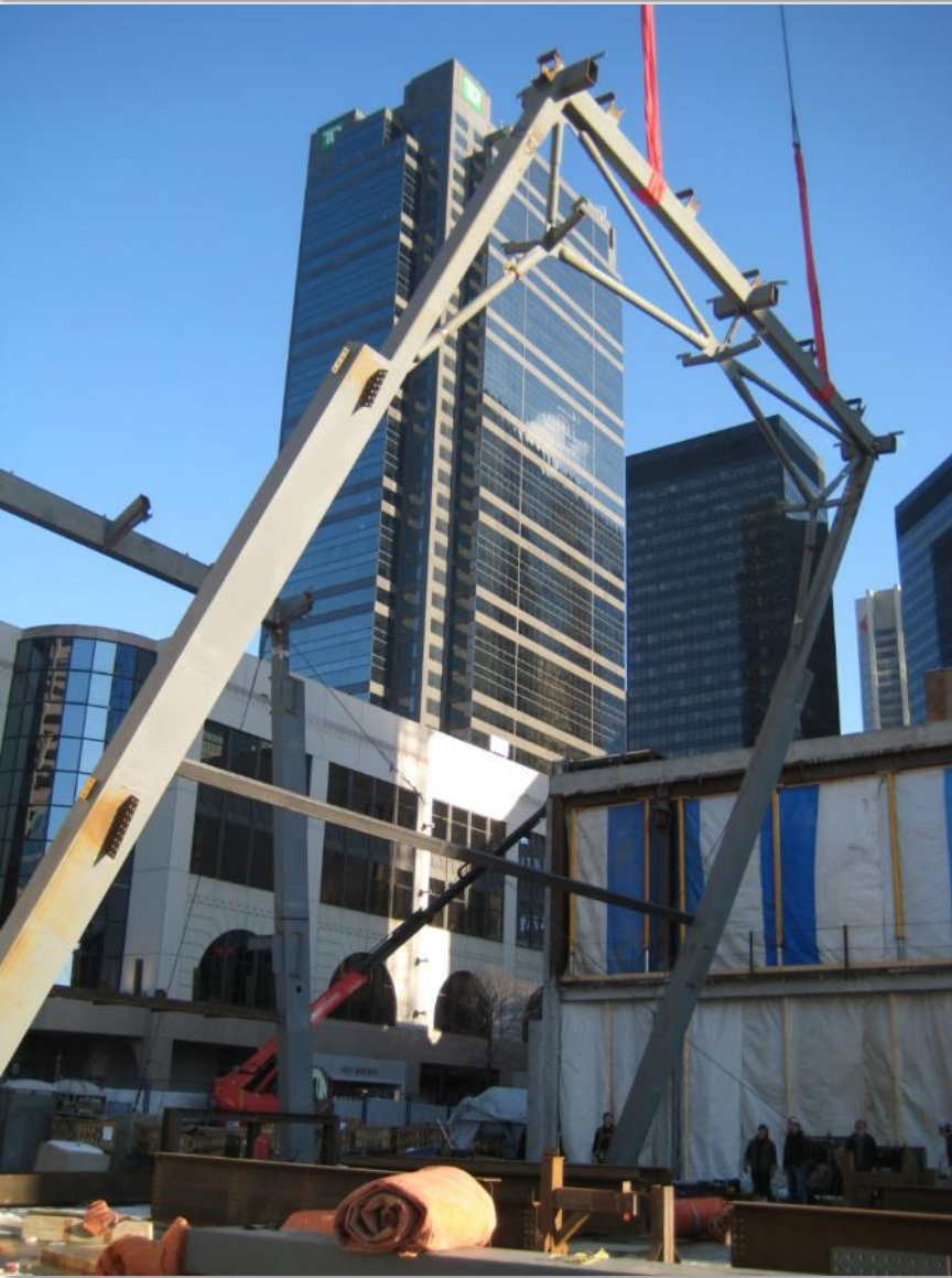
2 nd Arch erection
