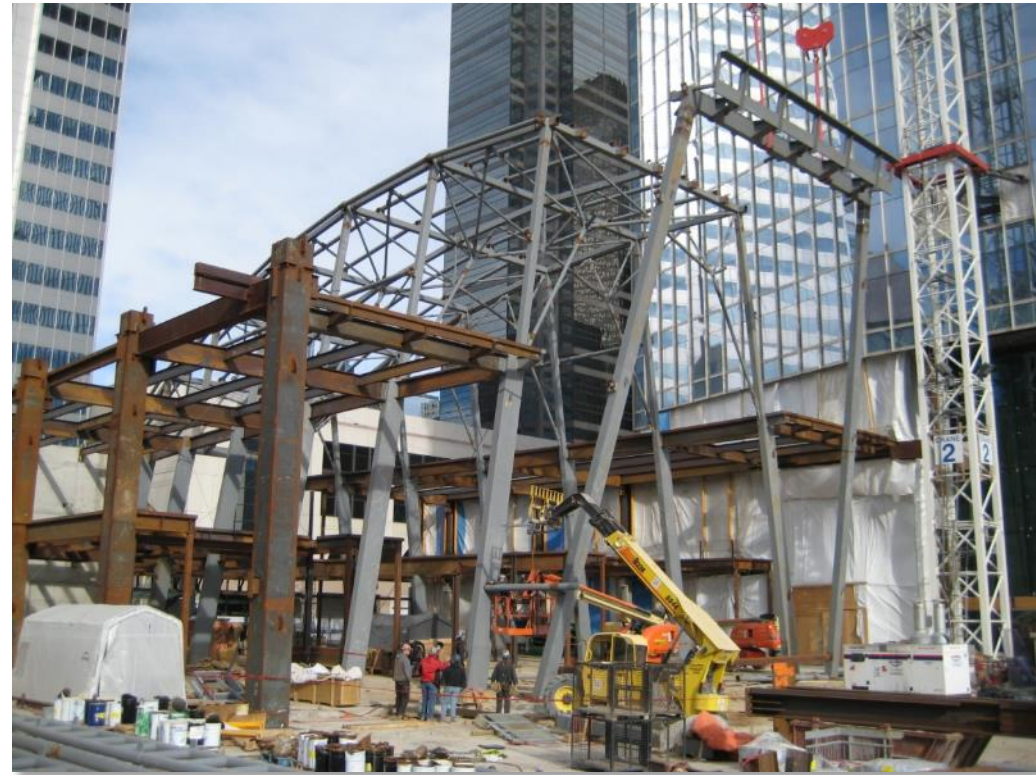
Last Arch erection
