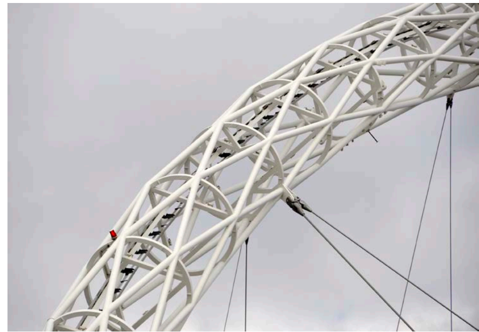
A protected ladder for access for servicing. Lift truck gets you to the access height.
