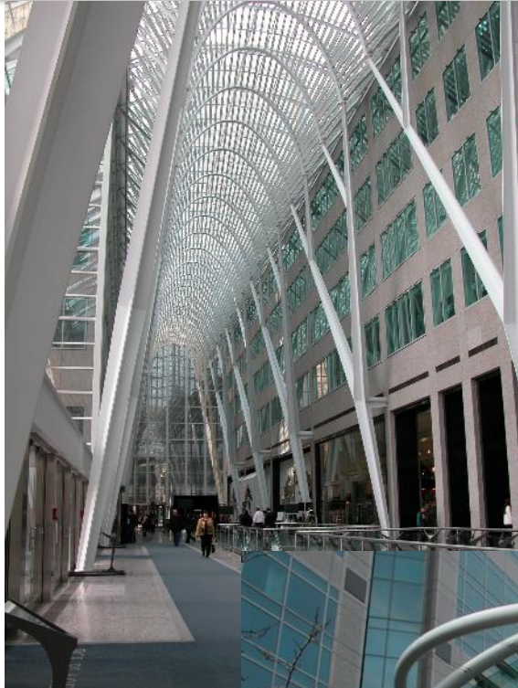
Custom platework + sharp edges
