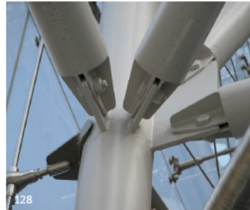
128 Tubular members can be connected using very inventive means. This combination of plates allows for constructability, minimal on site welding and enhanced interest in appearance.
