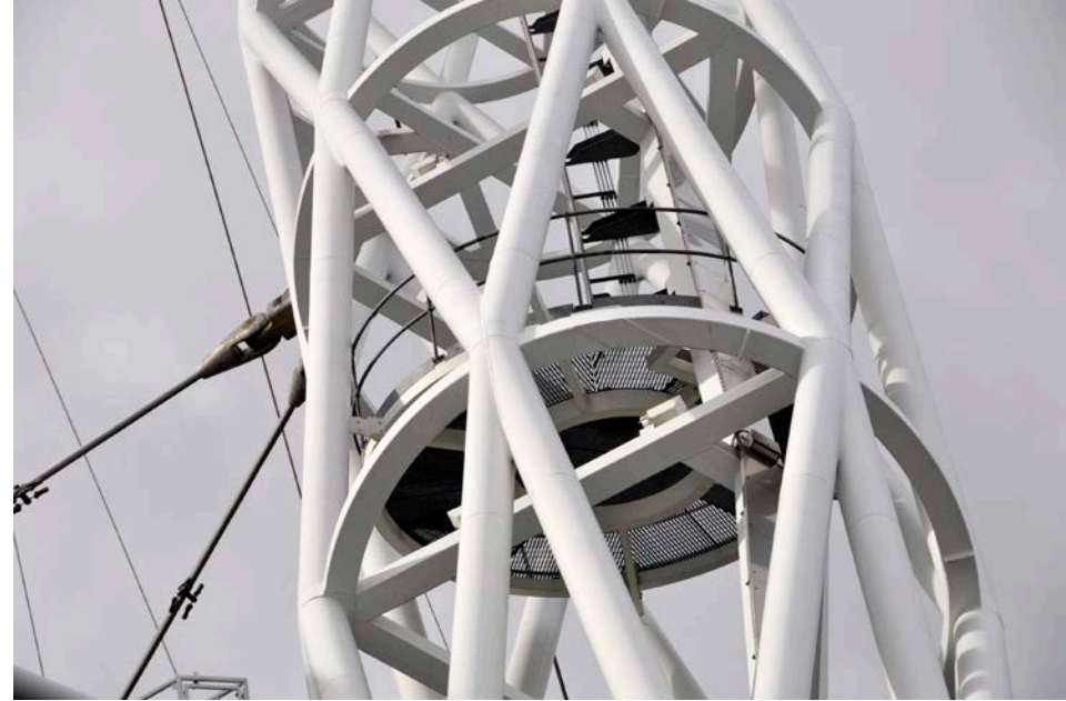
A protected ladder for access for servicing. Lift truck gets you to the access height.
